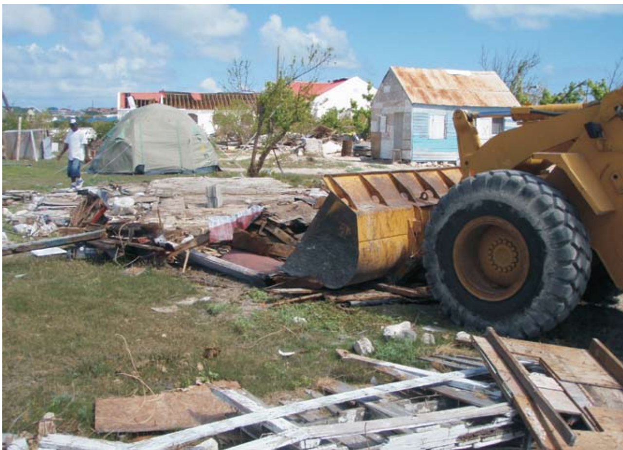
Clearing hurricane debris in post-hurricane Turks and Caicos Island 2008. Note the lack of appropriate equipment to segregate roofing and reusable boards. Source: MSB and Anttilator
