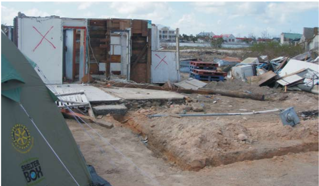
Typical hurricane debris where roof has been blown off and debris spread over area in post-hurricane Turks and Caicos Island 2008. Source: MSB and Anttilator
